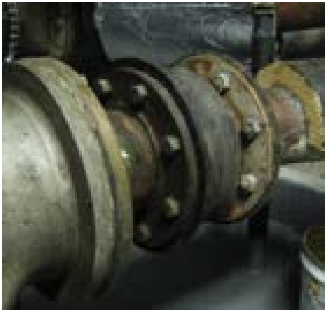
Figure 27: Example of a Fitting – a Flange
